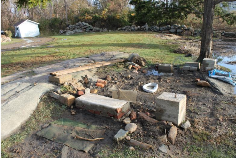
A sobering site: the Beach House was swept off its foundation by a midnight tidal surge.
