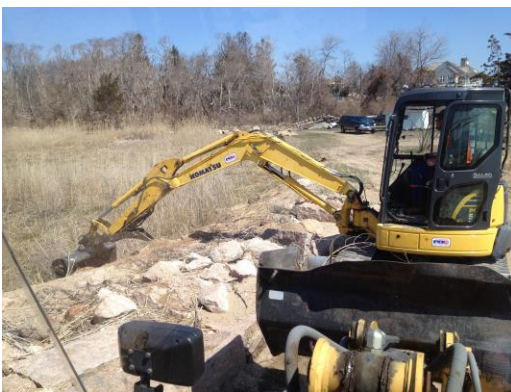
Todd Chemacki running the excavator.
