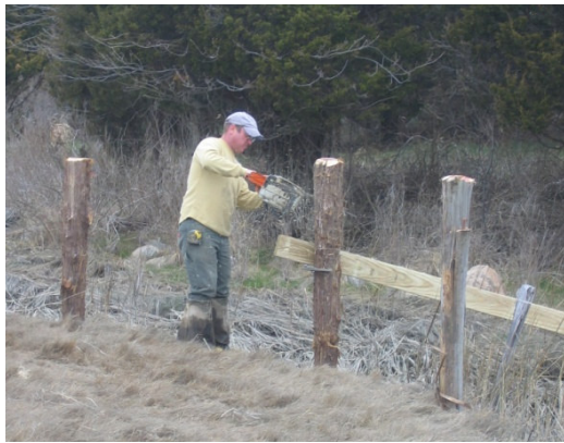
Eliot Benton installs a cross-brace.
